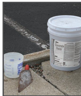
Concrete Patch (pg. 68)
